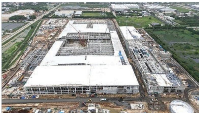
Bird's-eye view of the Micron SEZ "Pioneer" under construction at Sanand, Gujarat
